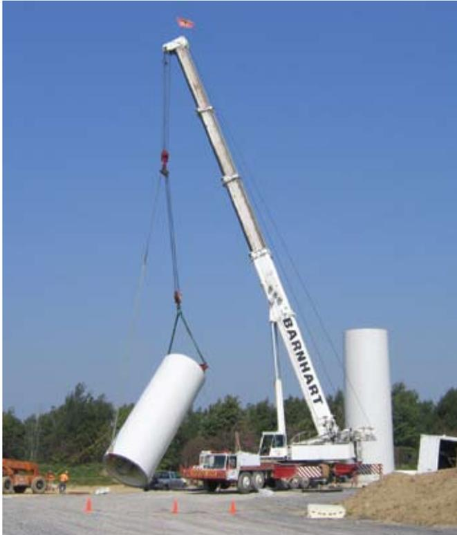
A state-of-the-art rigging system allows a single crane to pickup an angled load that usually requires two cranes. [Courtesy of Barnhart Crane & Rigging].
