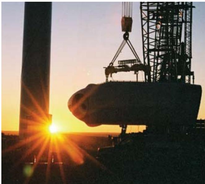
**Wind turbine nacelle installation. The nacelle weighs about 110,000 pounds and is the size of a school bus. [Courtesy of Barnhart Crane & Rigging].**
